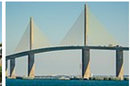
Sunshine Skyway Bridge
